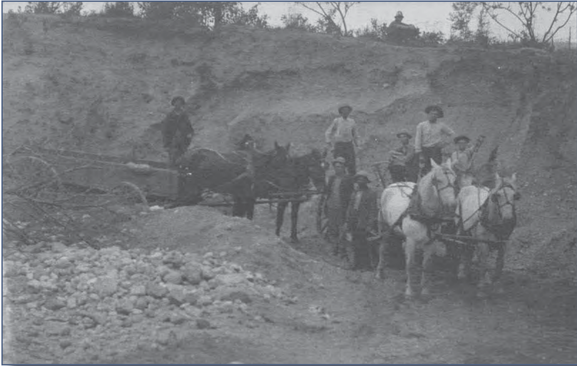
4.7: Building M-22. Photo: Arcadia Area Historical Society
